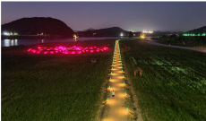
Installation of board lighting on the walkway
